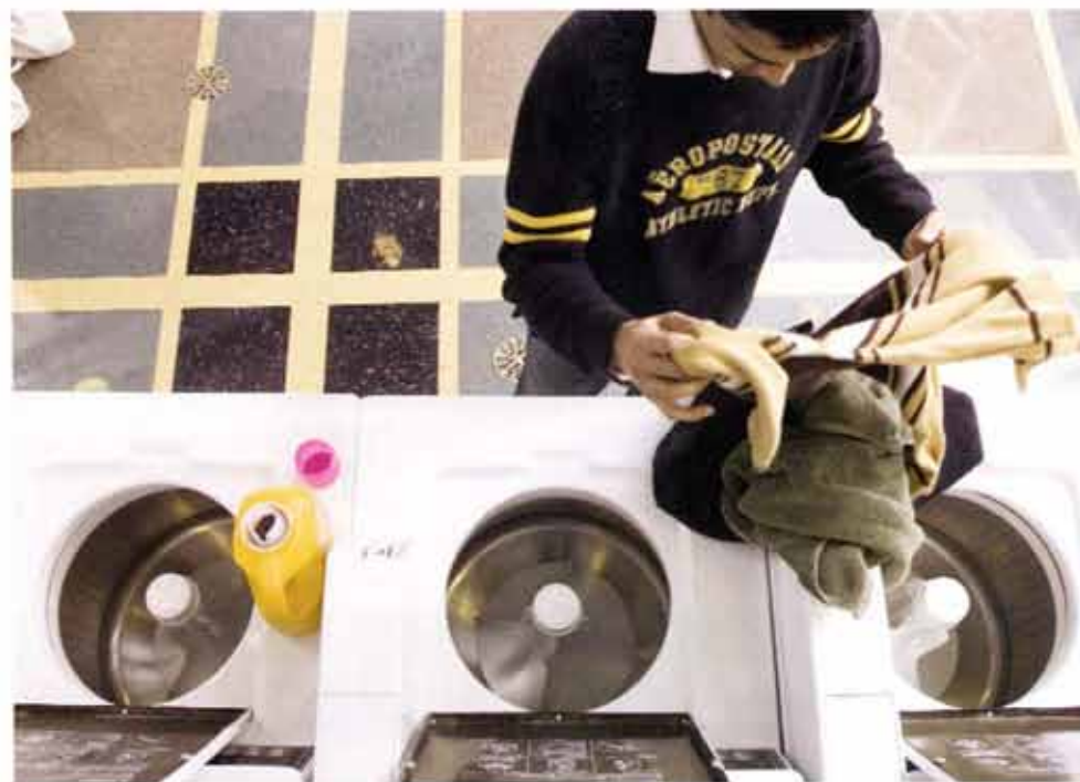
Laundry rooms like the one at Purdue University in West Lafayette, Ind. (above), must comply with the new Department of Energy standards, which took effect Jan. 1, 2007.
